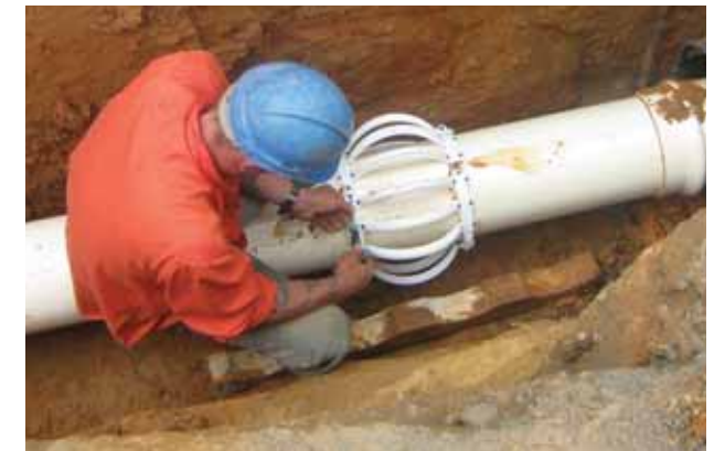
HD-75 being used on a 250mm OD pipe for a sewer installation in Queensland.
